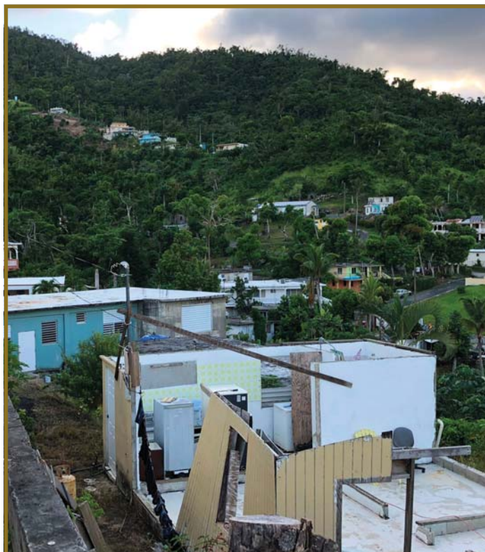
After nearly a year, much of the damage caused by Hurricane Maria remains. Photo by Lisa Cosby.
